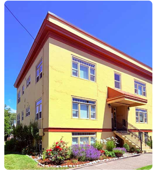
The Verna Vista apartment building was built in 1924
